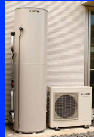
Heat pump hot water
