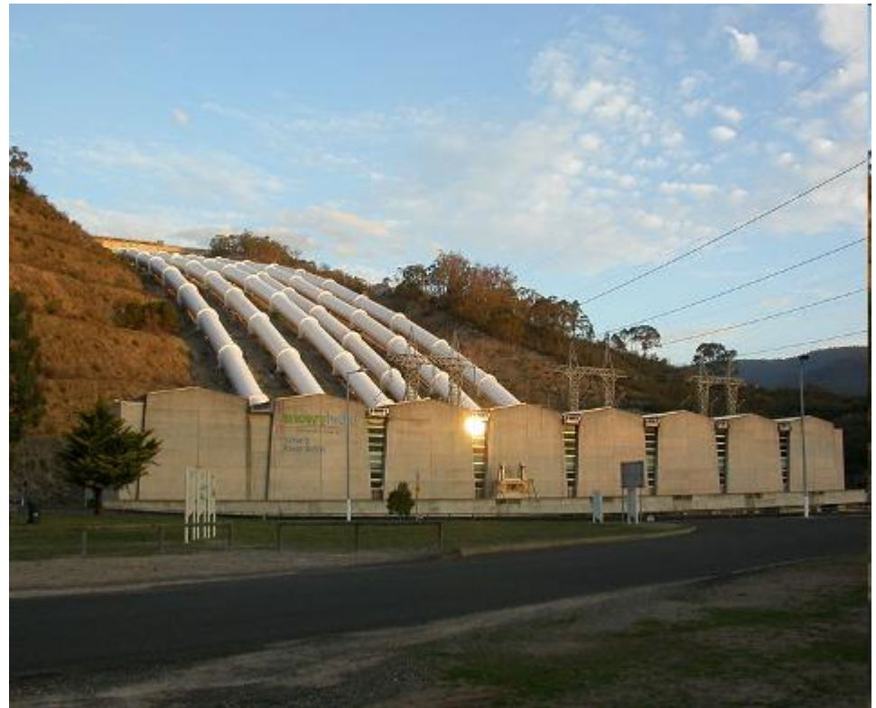
Tumut 3 1500 MW pumped hydro storage system in the Snowy Mountains © A Blakers
